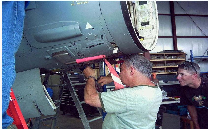
Pete and Mike are removing lots of rivets to make way for a new sheet metal repair.
